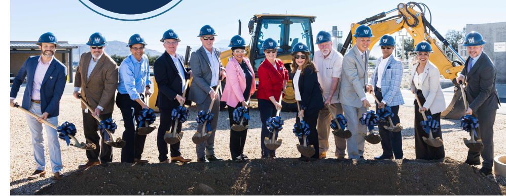
Western Water breaks ground on key infrastructure upgrade serving March Air Reserve Base and the region.
