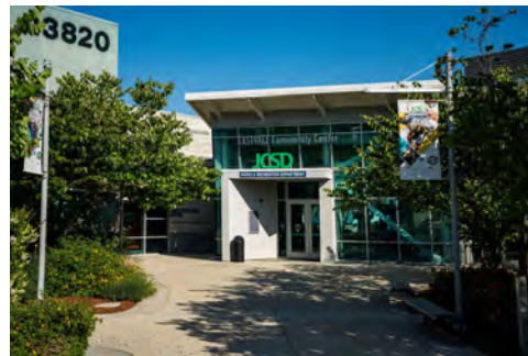
Eastvale Community Center, Eastvale
