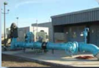
*Well 23 is located at JCSD's main facility on Harrel Street. The well was drilled in 2004 and produces 3505 gallons of water per minute.*
