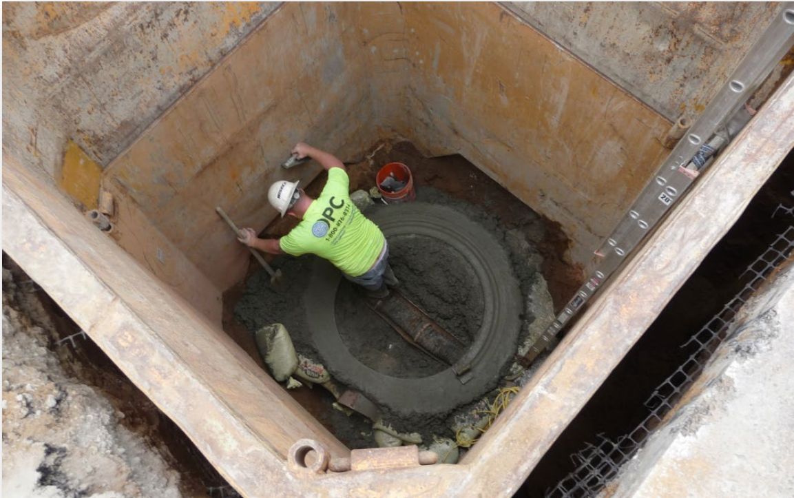
Manhole construction during JCSD's Florine Lift Station capital improvement project
