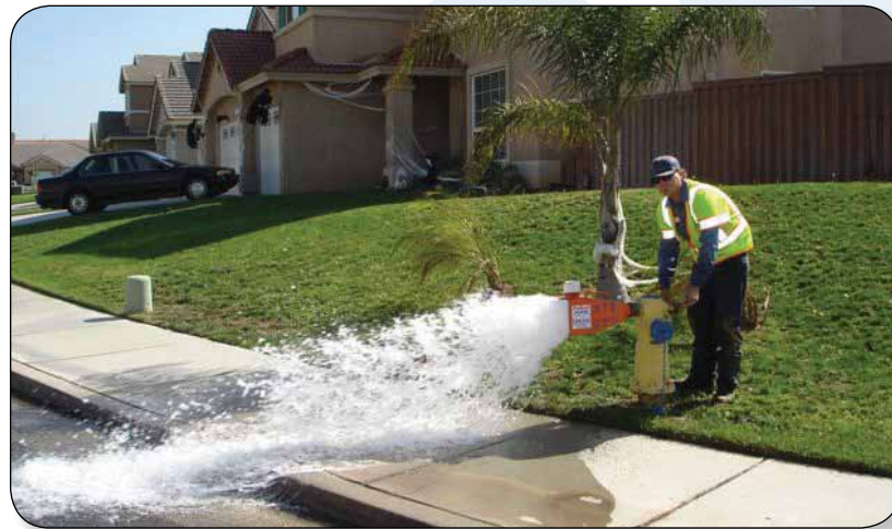
JCSD Water Service & Maintenance worker Todd Crowe flushes a residential hydrant.
